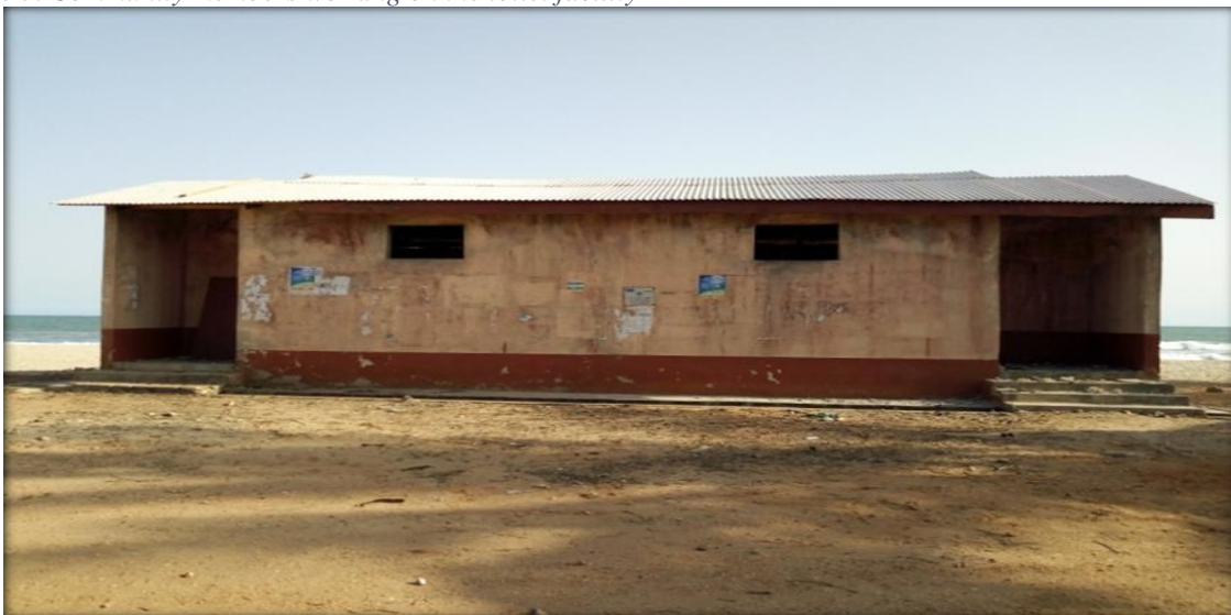
Figure 8. The refurbished toilet facility in Woarabeba community
