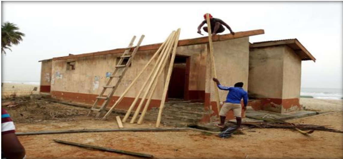
Figure 7. Community members working on the toilet facility
